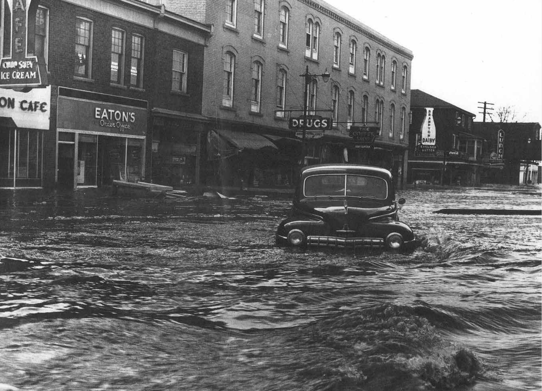
Brampton Flood, March 1948. Photograph by Russell K. Cooper. COURTESY REGION OF PEEL ARCHIVES.
